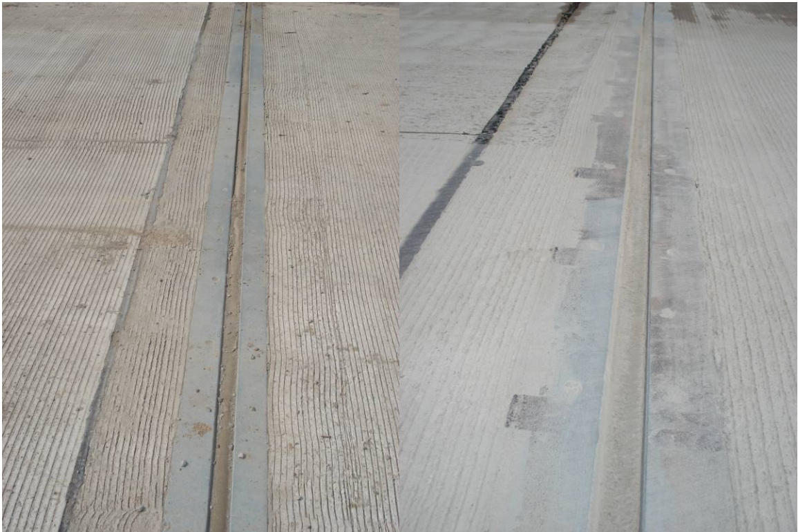
Figure 21: Shilcott Creek Bridge - Original Joint (left) vs. Replaced Joint (right)
