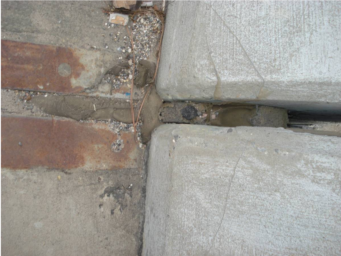
Figure 25: Pecan Street Double Backer Rod in Joint
