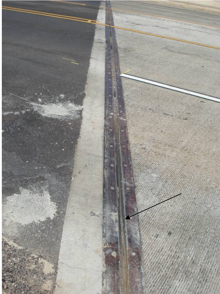
Figure 35: Blossom Way Creek Joint with Sealant at Roadway (8-14-07)
