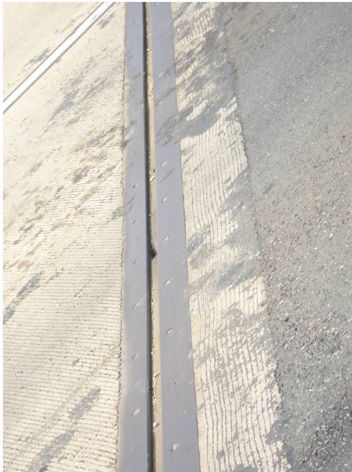
Figure 23: Grisby Ford Silicone Puncture
