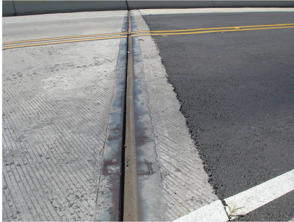
Figure 17: Mill Creek Road Bridge Deck Joint
