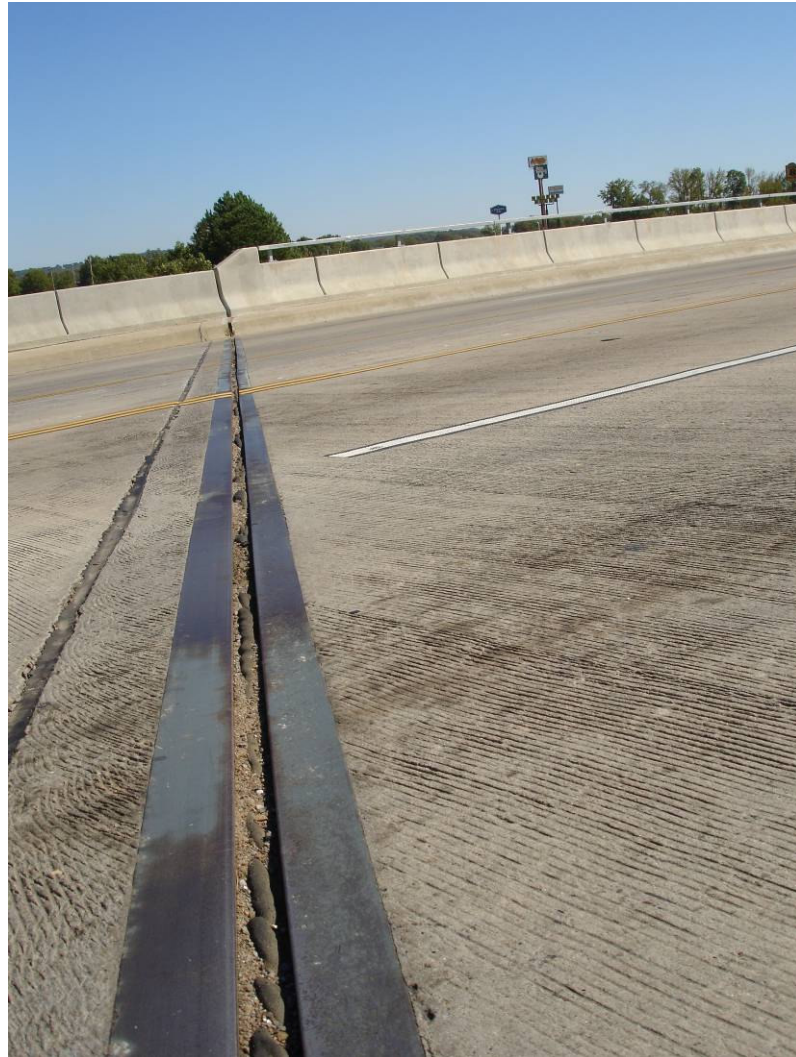
Figure 18: Highway 7 over I-40 Bridge Deck Joint
